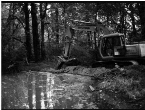
Figure 633-1. David Parker makes a dam at Mtn Grove with an excavator
